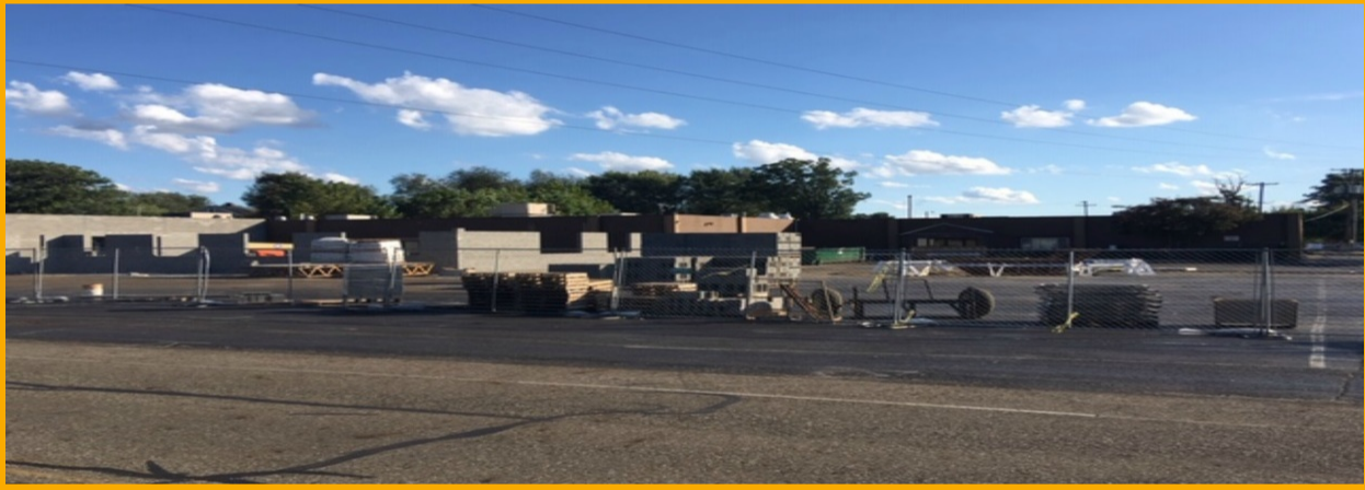
JRC Campus at Meyers Lake under construction
